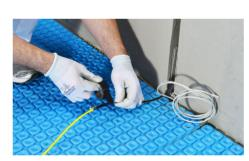
1. Installing cold tails and floor temperature sensor Insert the cold tail and temperature sensor(s) into the conduit from the base of the wall up to the thermostat electrical back box
