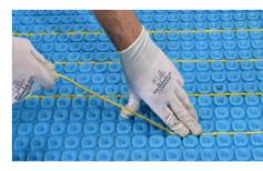
2. Install heating cable in the membrane Press the ThermoSphere heating cable into the membrane using a float or roller. Observe the recommended spacing of 3 dimples for 130W/ m<sup>2</sup> and 2 dimples for 195W/m<sup>2</sup>. Take care not to damage the cable.
