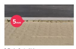
3. Check adhesive thickness According to building norms, heating cables must be covered with a 5mm layer of adhesive as a minimum. Check that your adhesive layer complies
